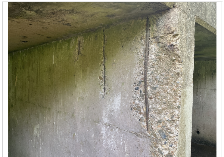
Spall with exposed rebar at inlet end of divider wall.
