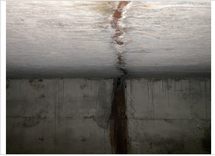
Cracks with efflorescence and rust staining in barrel 1.
